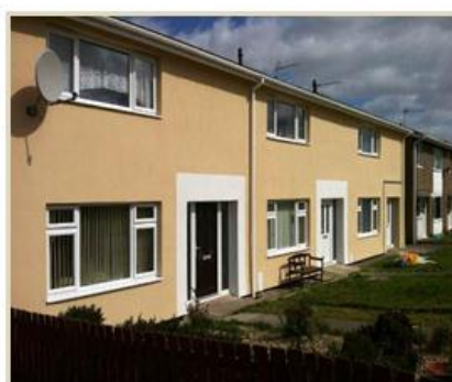
Radburn Estate , on completion
